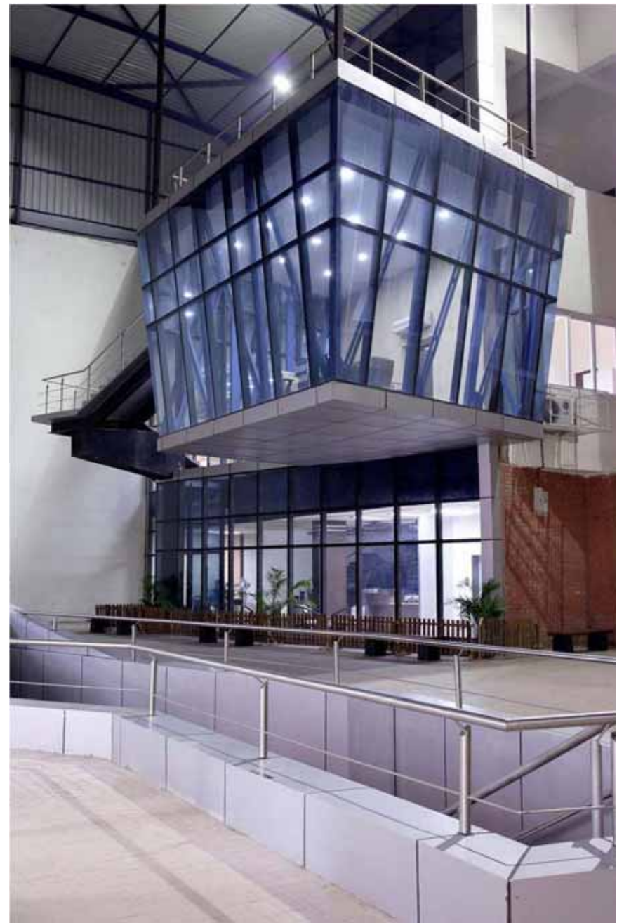
view of cantilevered principal's cabin
