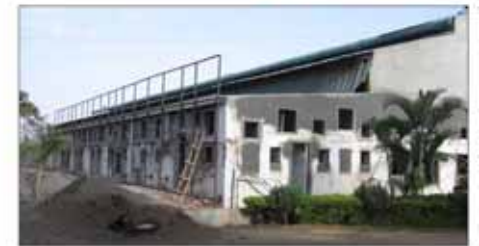
ongoing site construction_10th May 2008.
