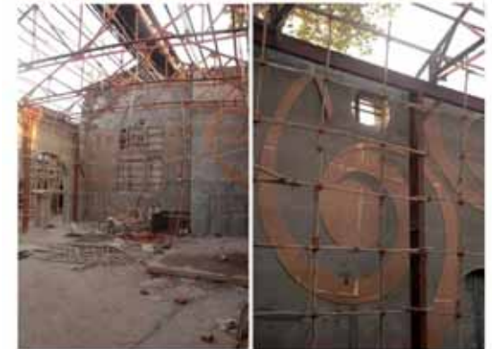
Under construction pictures
