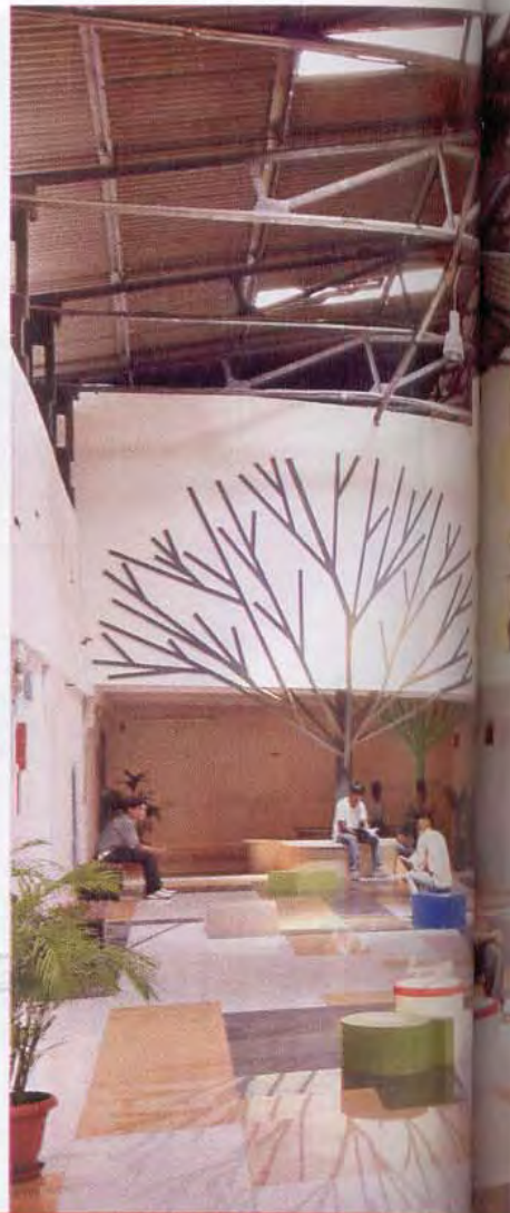
They gutted the core and put in a mezzanine supported on an independent steel structure. The partitions and
