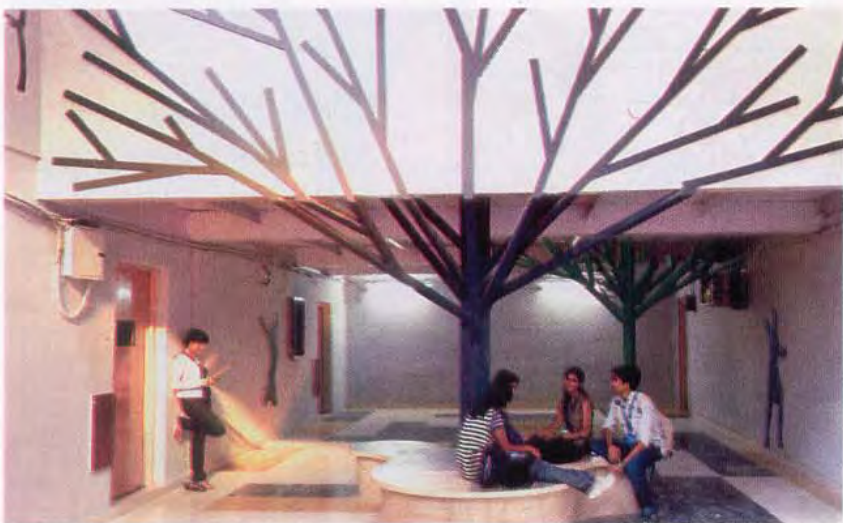
They gutted the core and put in a mezzanine supported on an independent steel structure. The partitions and
