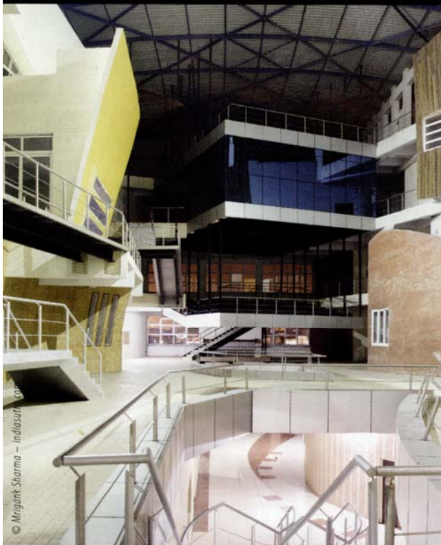
Principal's cabin – one of the most exciting parts of the whole project. Hung from the roof trusses by the help of steel cables enables the head of the institution to keep an eye on all the activities happening down below.
