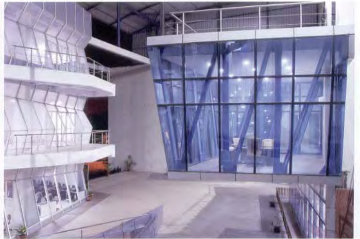
View of administration block
